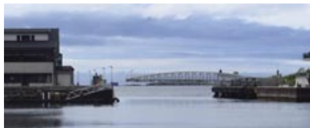
Pedestrian swing bridge, Fosnavåg, John Sadd
